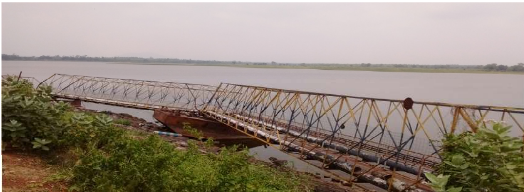
Sali reservoir and the raw water main
